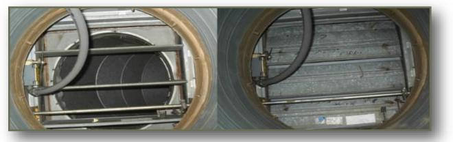
A thorough inspection is required by NFPA to ensure a fire damper is properly maintained and in working order to stop the spread of a fire. Upon inspection, the building management must be provided a detailed report of every fire damper.
